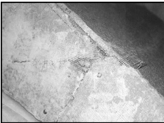
Sloppy cuts can be avoided by using either a four-inch diamond blade on a high-speed grinder, or a masonry blade loaded on a circular saw.
