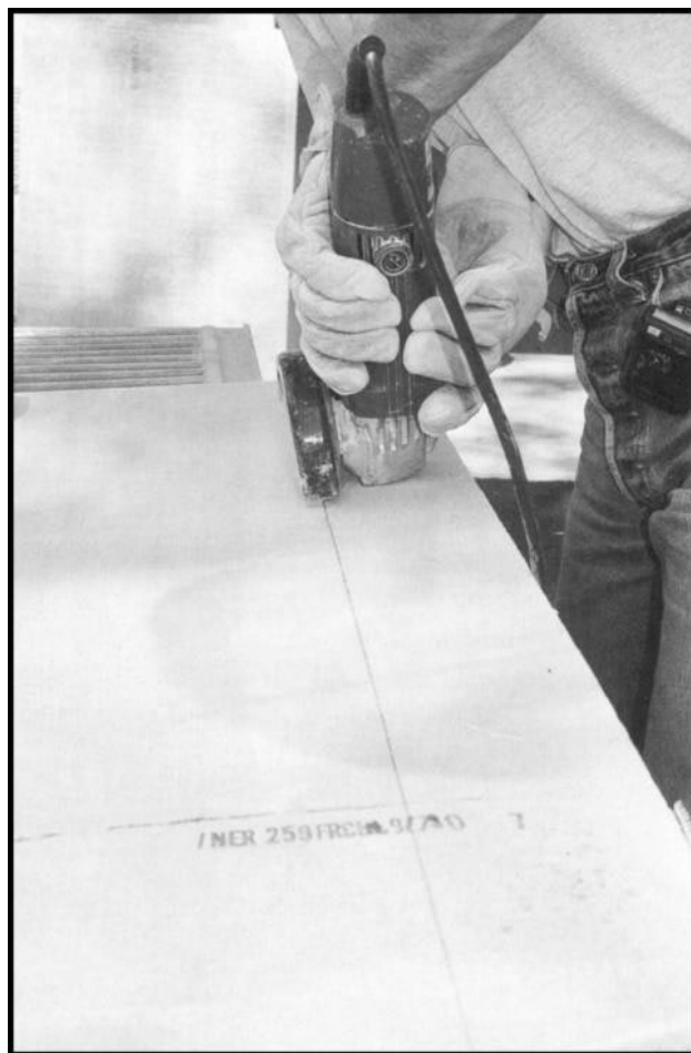
A four-inch diamond blade on a high-speed grinder is the best way to cut cementitious backer units. The tool can make any kind of complex cut.
